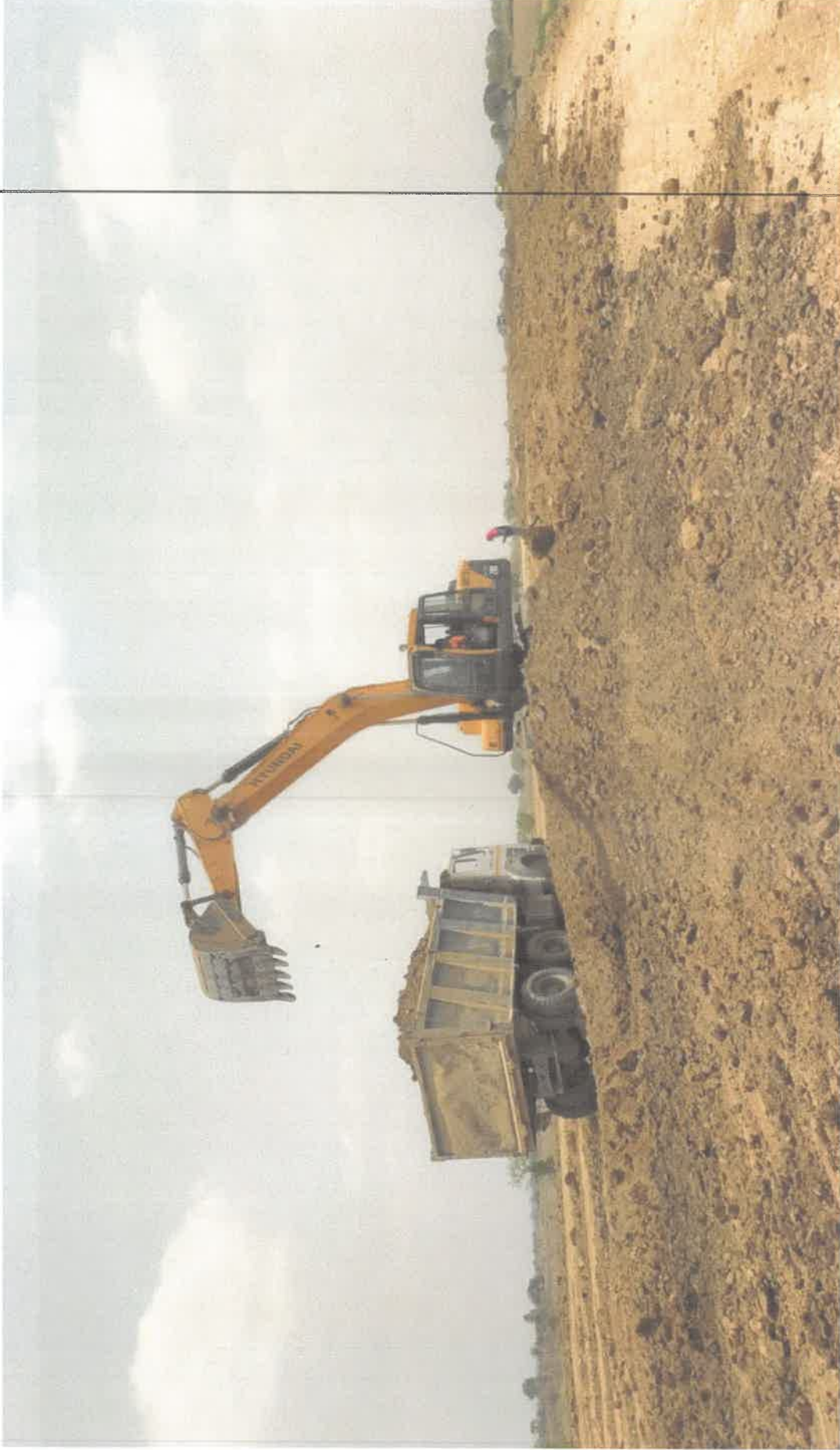
Black cotton soil removing at site
